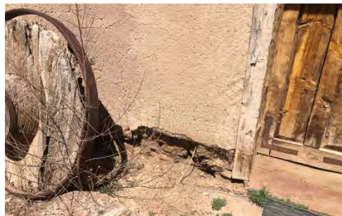
In the photo above, this courtyard image shows characteristic deterioration of walls at base on Romero House. At right, a view of the courtyard wall of Carson House, showing generally poor condition of exterior finishes and deterioration at base of wall.
