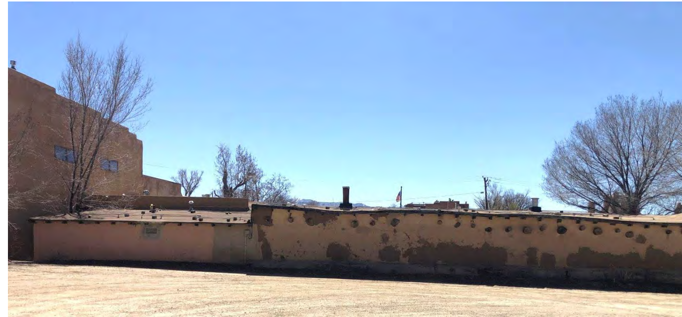
The photo above shows the north wall of Romero House. At left, a closer look at the mud plaster portion of the north wall, with the contra pared. Below, a look at the west wall of Romero House.
