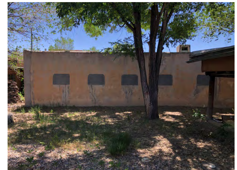
The photo above shows the north wall of Romero House. At left, a closer look at the mud plaster portion of the north wall, with the contra pared. Below, a look at the west wall of Romero House.
