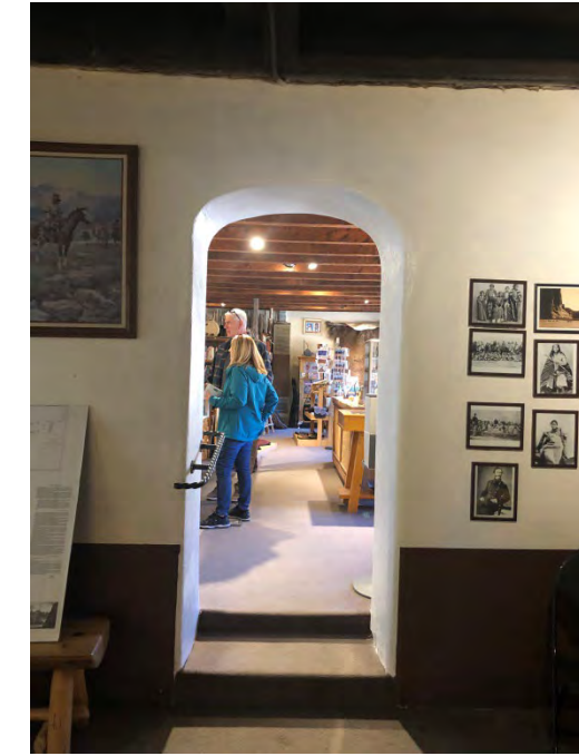
Top, door plan for Carson House. Above, two of the doors in Carson House.
