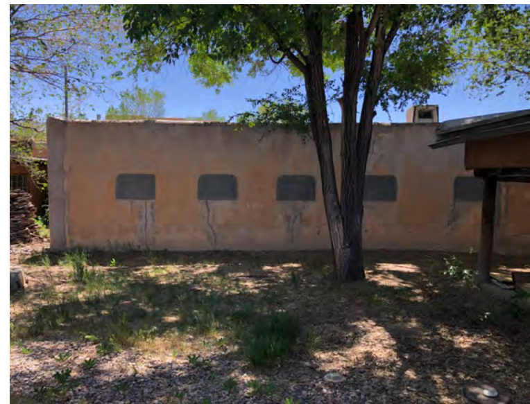
West side of Carson House, including in-filled windows at Carson Room 5 and gate at street.
