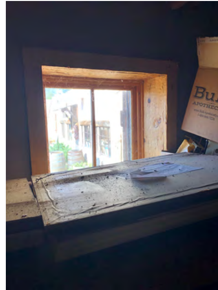
WINDOW 16 - AT ROOM 4
