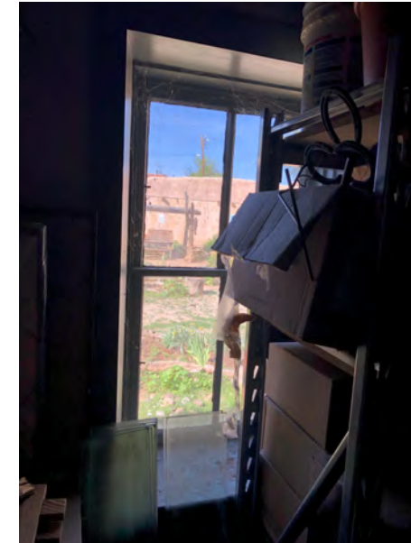
WINDOW 17 - AT ROOM 3
