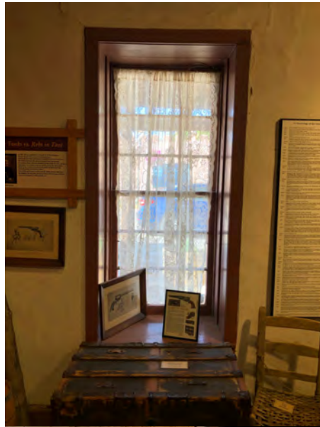
WINDOW 1 - AT ROOM 1
