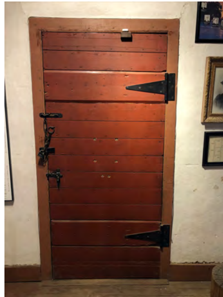
DOOR A - INTERIOR
