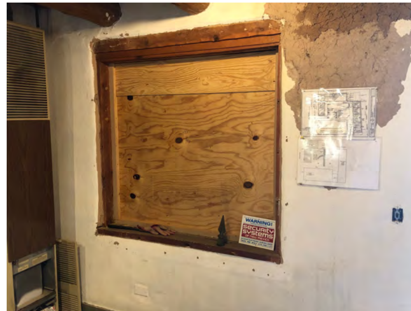
WINDOW 19 - AT ROOM 1
