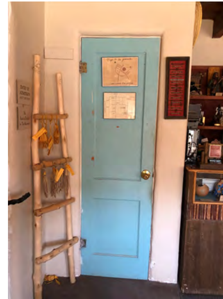
DOOR I - AT ROOM 5
