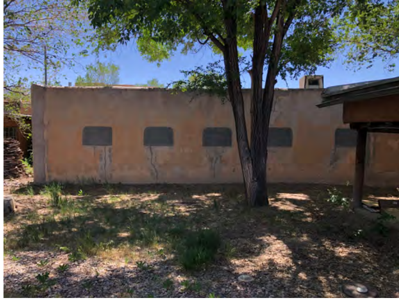
WINDOWS 11-15 - EXTERIOR (WINDOWS INFILLED - ONLY VISIBLE OUTSIDE WEST WALL)
