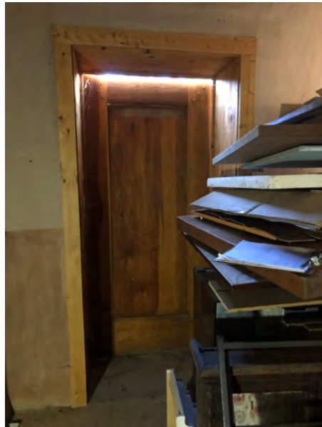
DOOR J - AT ROOM 4
