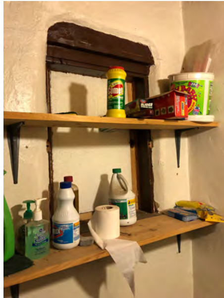
WINDOW 20 - AT ROOM 1
