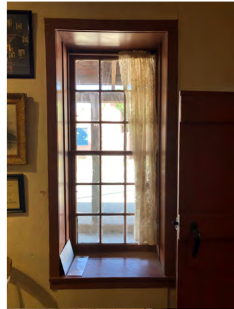
WINDOW 2 - AT ROOM 1
