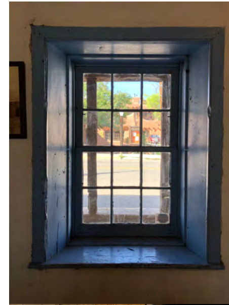
WINDOW 3 - AT ROOM 2
