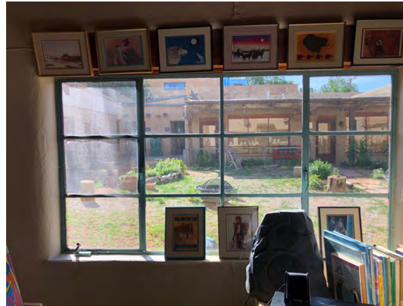
WINDOW 10 - AT ROOM 5
