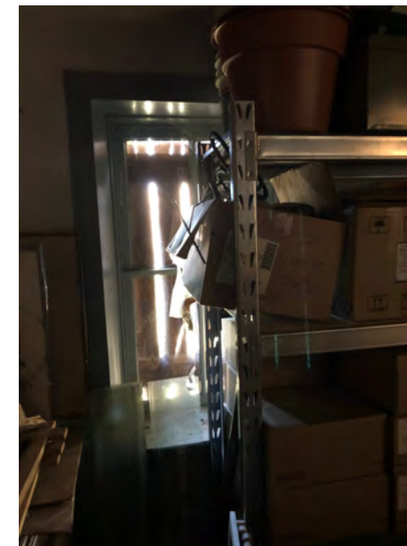
WINDOW 17 - AT ROOM 3
