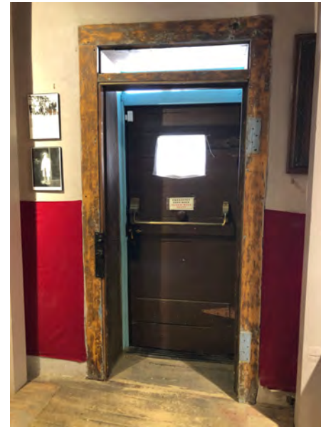
DOOR D - AT ROOM 3
