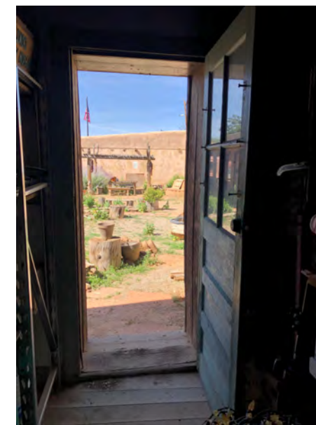
DOOR K - AT ROOM 3
