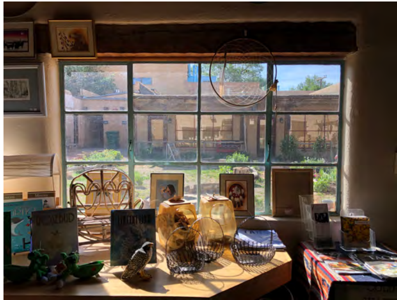
WINDOW 9 - AT ROOM 5
