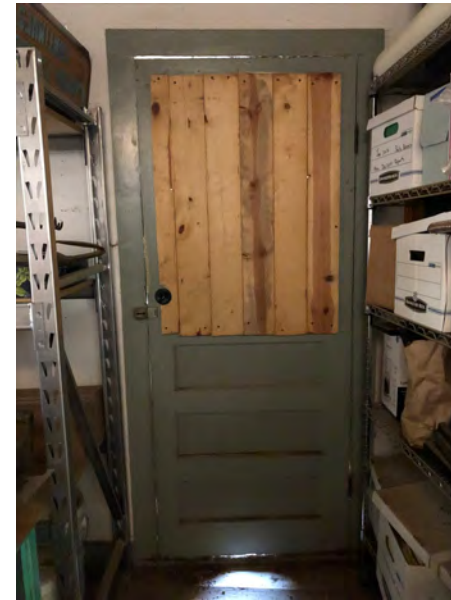
DOOR K - AT ROOM 3
