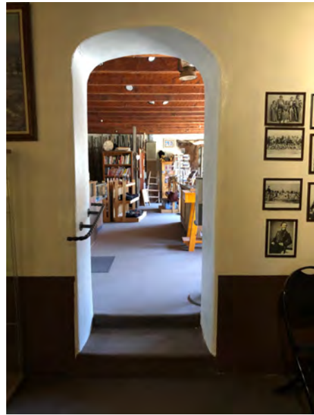
DOOR F - FROM ROOM 4
